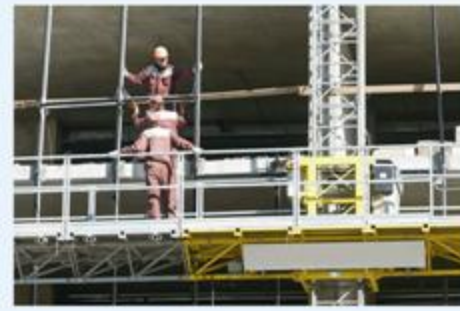
Working on worksite
